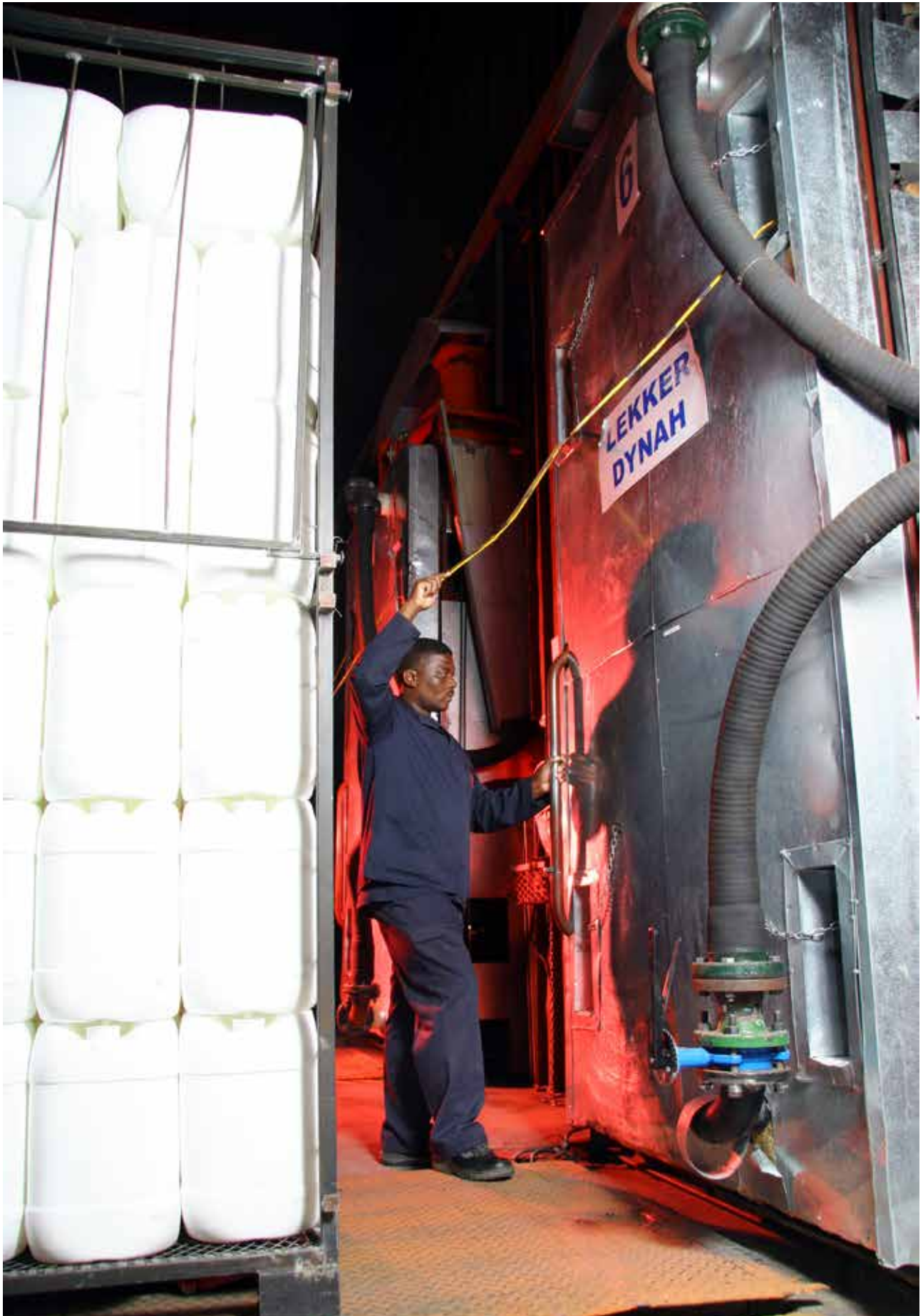
Pelchem Surface Fluorination Plant
